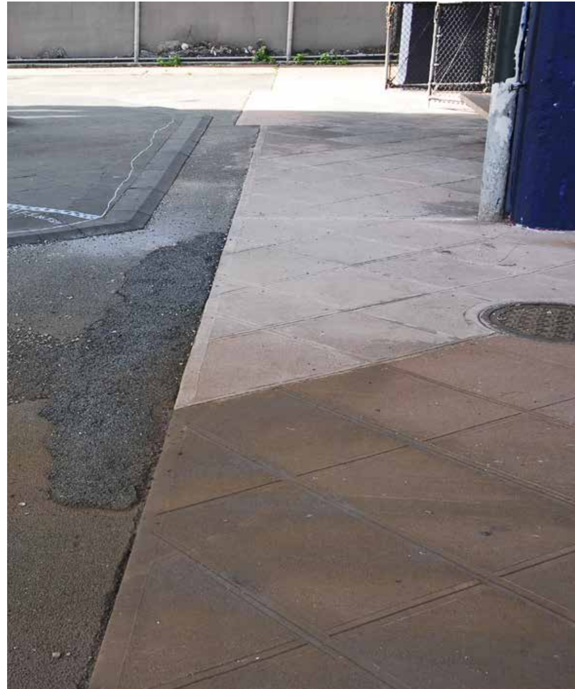
2. SUNLIGHT REACHING GROUND PLANE UNDER OVERPASS
