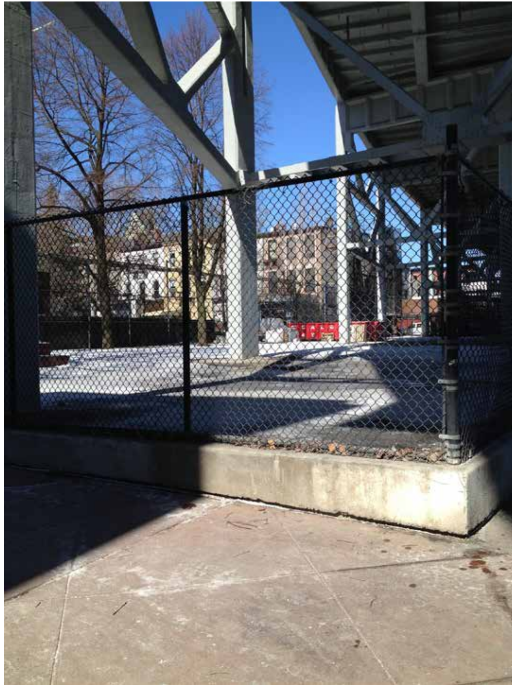
1. SUNLIGHT REACHING GROUND PLANE UNDER OVERPASS
